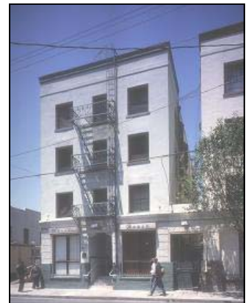
The Marshal House's roof and kitchen will be upgraded and a new elevator will be installed.
